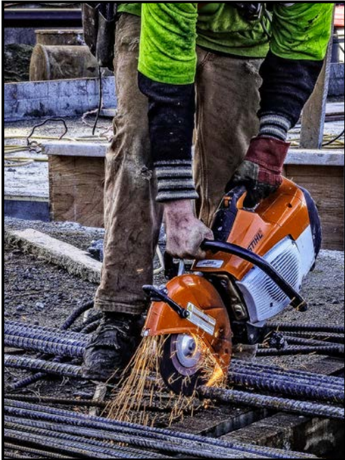
"Cutting Rebar"
