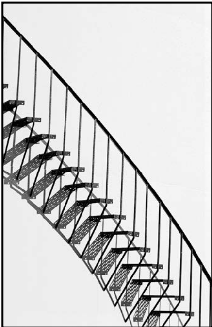
“Stairs”, Texaco Tank Farm, Kingston St., Victoria, 1983
